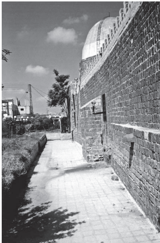
FIGURE 8 The decorated floor reburied below the pavement.
