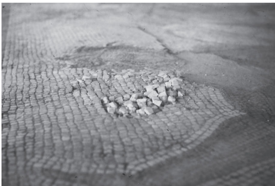
FIGURE 3 Aizanoi, Roman bath. Detachment of tesserae (1994). Photo by Y. Selçuk Sener.
