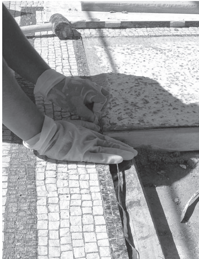
FIGURE 3 The mosaic reproduction. Lead strips were mounted to separate the main figures from each other, as in the original mosaic. Photo from Letoon Project archive with the permission of Dr. Didier LaRoche, Letoon project director.
