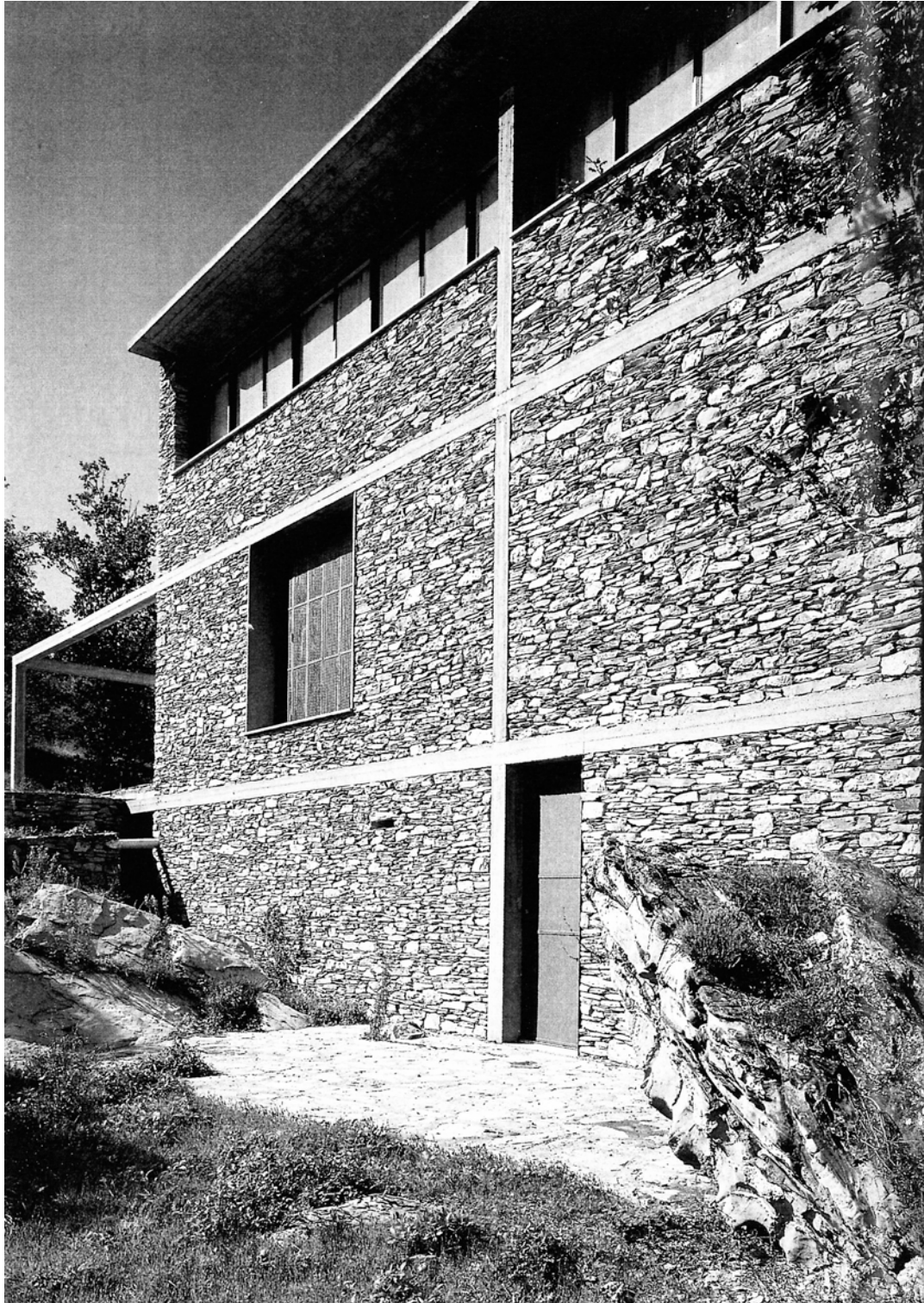
Figure Three – Stone House, Herzog and de Meuron
