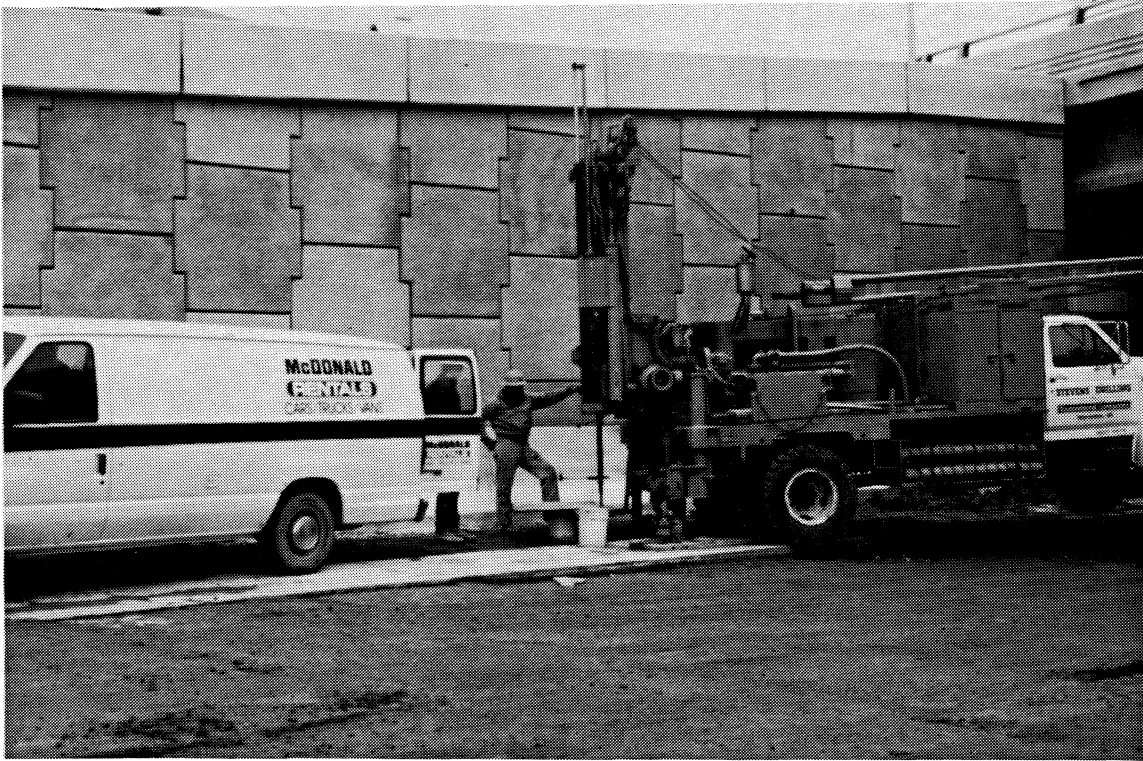
Figure 4.2. Piezocone Testing Operations at Port Huron, Michigan.
