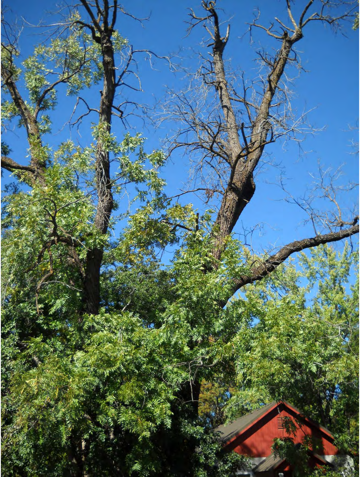
Walnut at 618 W 2nd Ave in the F:3 position. Tree is mostly dead and hangs over the house.
