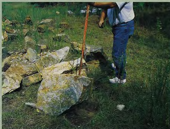
Top: Using a small stone as a fulcrum, a pry bar can be used to lift a rock up and change its position slightly. Above: Medium-size stones can be moved short distances by “rolling” them end over end with a pry bar.
