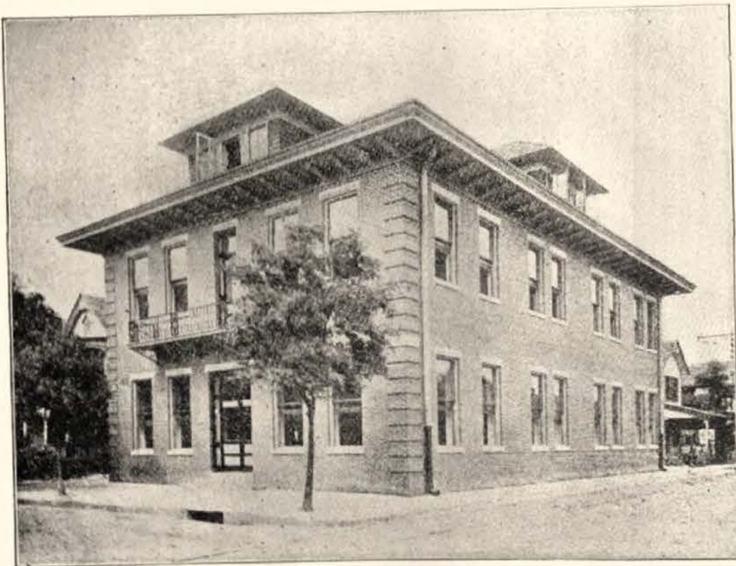
State Board of Health Building, Tampa, Florida.
